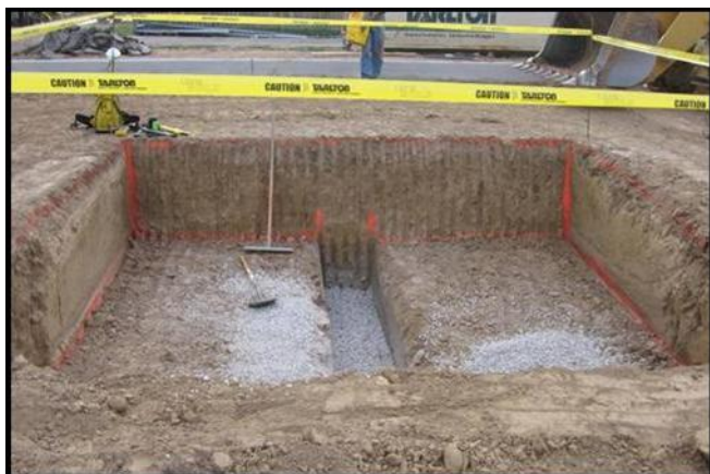
Figure 1. GPR test area, pit excavation prior to placement of pipes.
