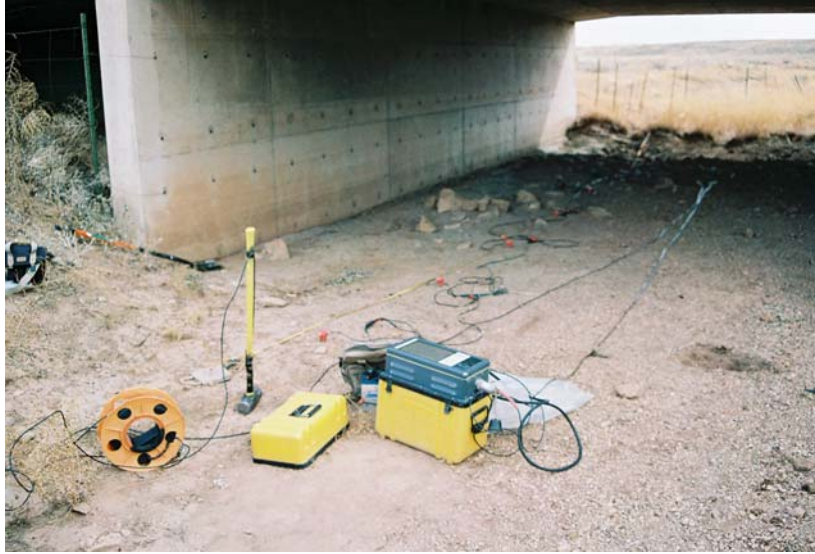
Figure 9. Surface seismic setup under bridge. Unlike the typical channel upstream, considerable coarser material was exposed at the surface under the bridge. The tops of the pier footings were generally exposed under the bridge but were covered at ends of the piers. The channel bottom appeared to be several inches higher than the tops of the footings; the ground surface grade and sloped to the footings.
