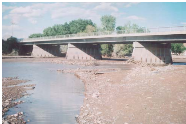
Figure 1. Beaver Dam Wash Bridge (Piers 2, 3 and 4) in Northwest Mohave County, Arizona after winter 2005 flood. Surface seismic lines were completed between each set of piers and abutments. Surface resistivity was completed at a previously installed piezometer on a gravel bar in the northern portion of the stream channel bed.
