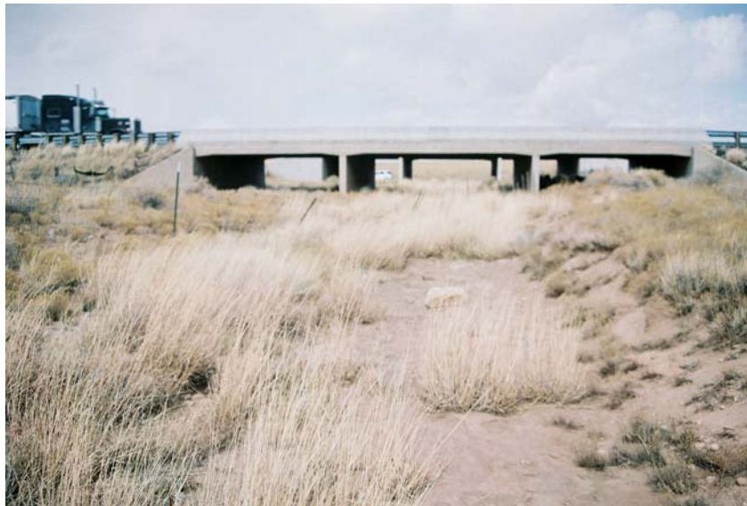
Figure 8. East-bound Babbitt Tanks Wash Bridge is in foreground looking north. Piers 1 and 2 are located in or adjacent to the active channel of Babbitt Tanks Wash. Based on the 1944 plans, pier foundations are three-foot (0.9 m) wide strip footings that are 18 inches (0.46 m) thick. Plans showed footing bottoms set approximately six inches (0.15 m) below the "Probable Solid Rock Line."
