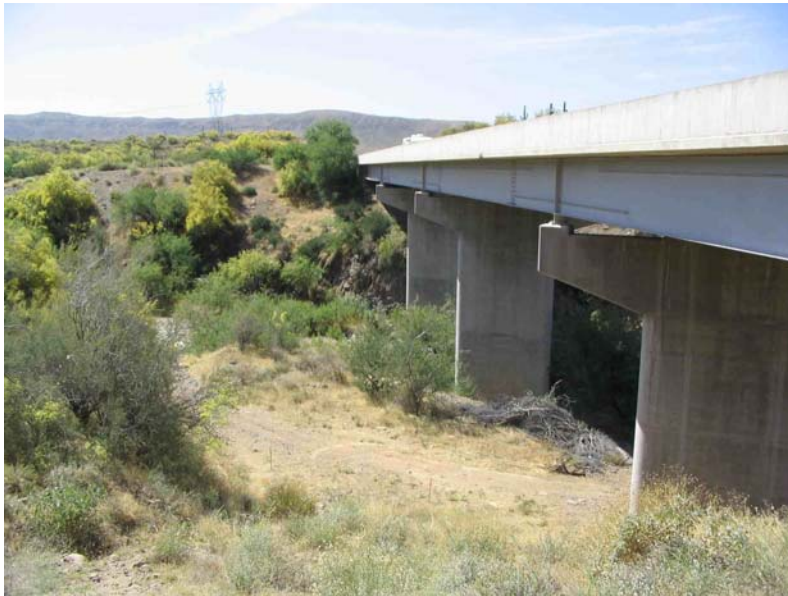
Figure 5. Little Squaw Creek Bridge, constructed in the 1960's, is a 2-lane, 5-span, 315-foot (96 m) long bridge constructed of reinforced concrete. The structure is supported on spread footings at both the south abutment and pier locations. Seismic lines were completed at or between Piers 1 and 2 in or near the active channel. Equipment was hiked into the small canyon from the vehicle parked by the highway.
