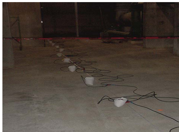
Figure 5: Geophones were placed inside sand bags and placed on top of concrete.
